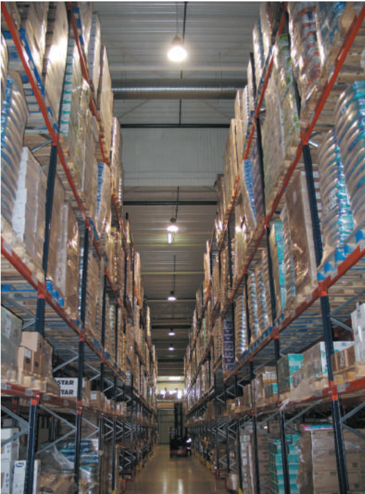
Highbay fittings with metal halide lamp and energy consumptions of 440W each before. Height 10-12 meters.
